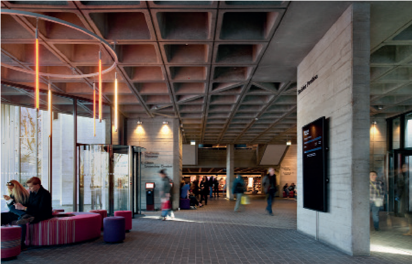
Left: Waffle slabs were used extensively in the 1960s, including on the National Theatre as these used less concrete for the same performance as a flat slab
